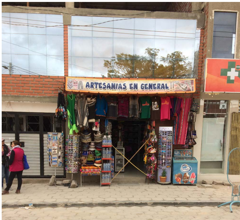
Figure 3. Future commercial gallery in the center of the city of Uyuni. Own source (2017)
